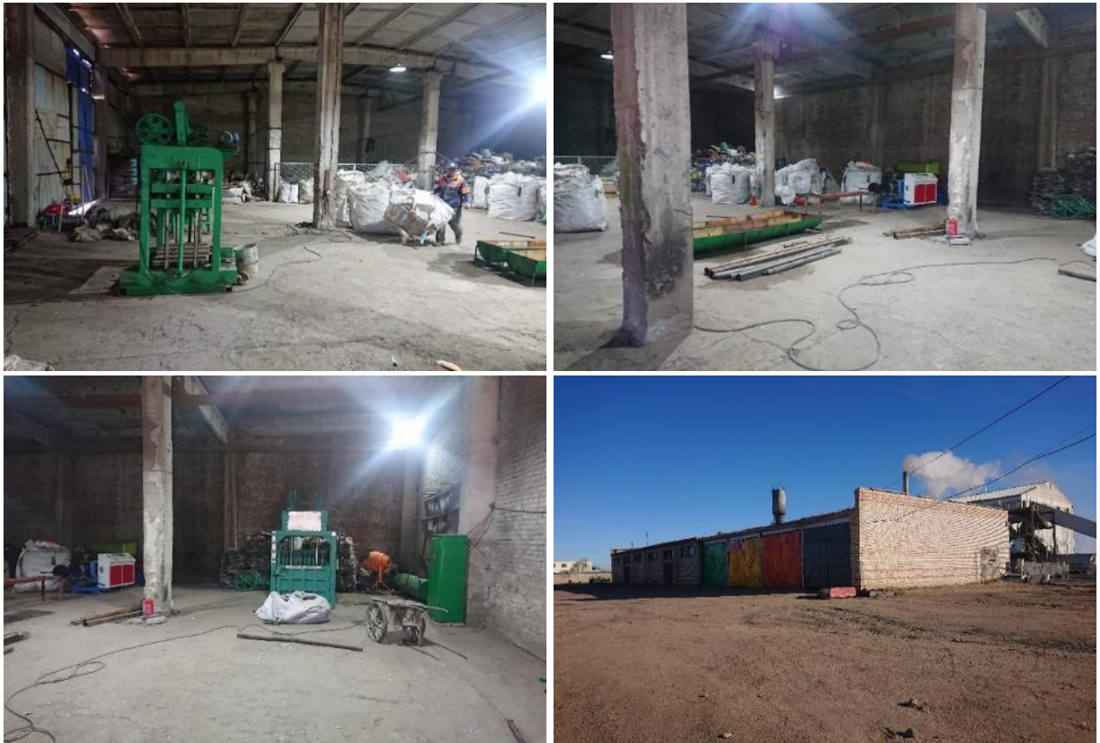
Figure 24. Solid waste recycling factory
