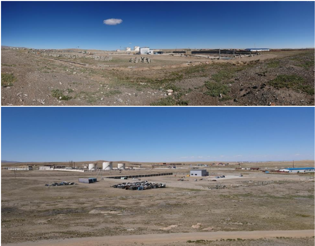
Figure 13. Solid waste transfer station with weighbridge
