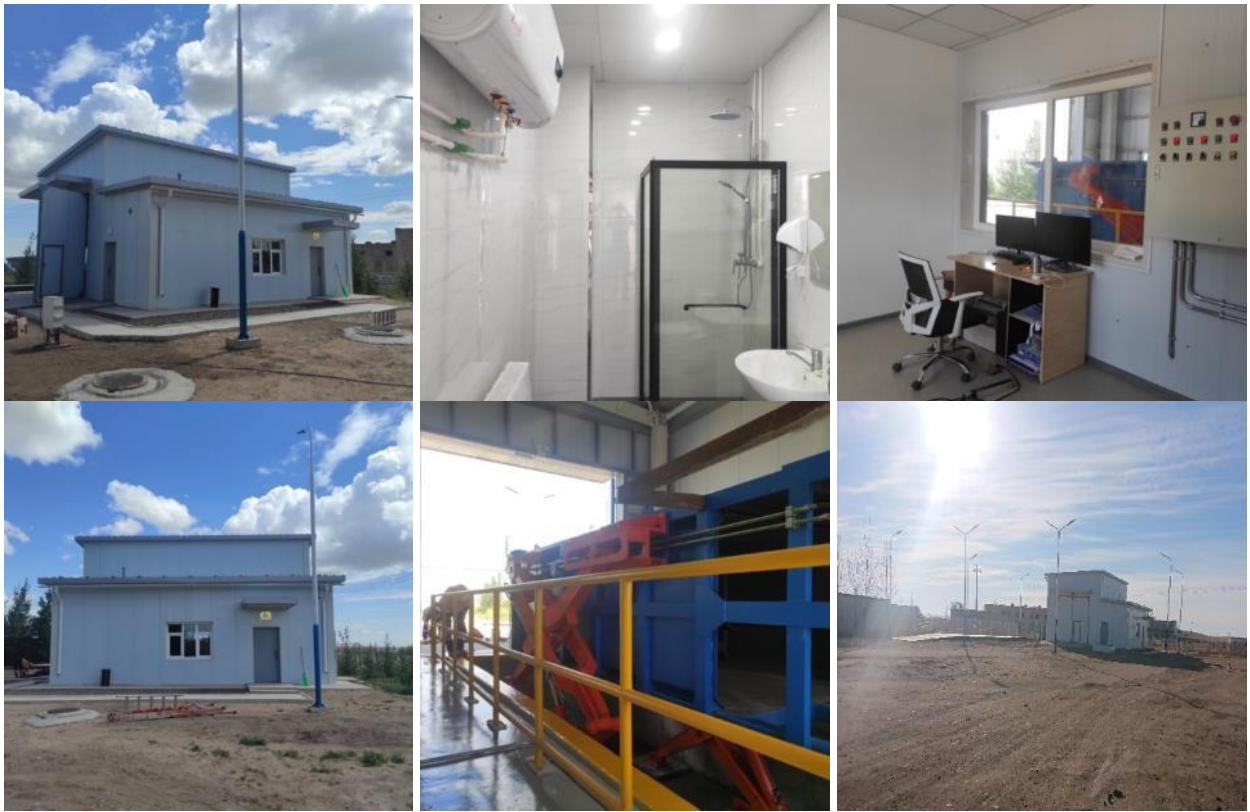
Figure 23. Solid waste compaction station and weighbridge
