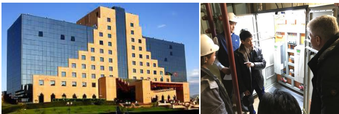
Chingis Khan Hotel and Two Inverters for Circulating Pumps
